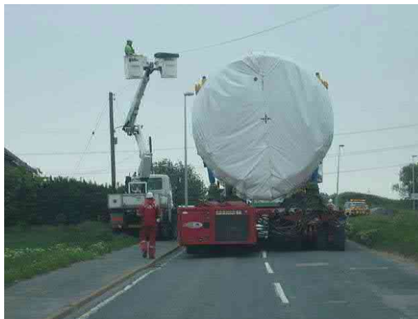
Source: Abnormal Load Engineering Library Photograph 2
